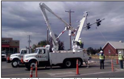
Public Works crews install the pedestrian crosswalk light on South Lincoln
